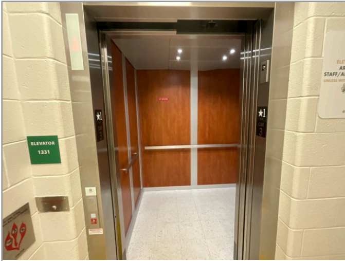
LOBBY LOOKING AT CABS
