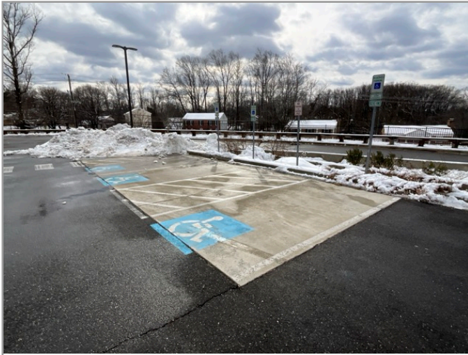
OVERVIEW OF ACCESSIBLE PARKING AREA
