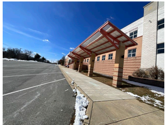
34 - BUS LOADING AREA
