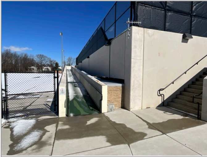
ACCESSIBLE ROUTE TO PLAYGROUND
